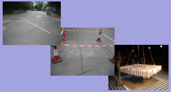
Saw cut and core drill to remove the concrete slab
