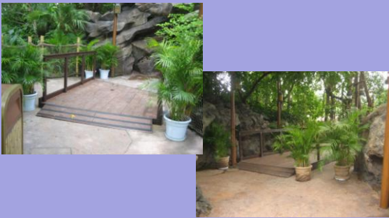
A wooden gangway to protect the newly laid concrete
