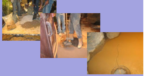
Laying of concrete and stamping concrete with mould
